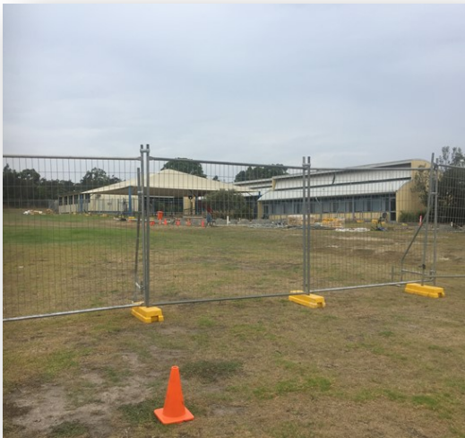
Fences in Place
